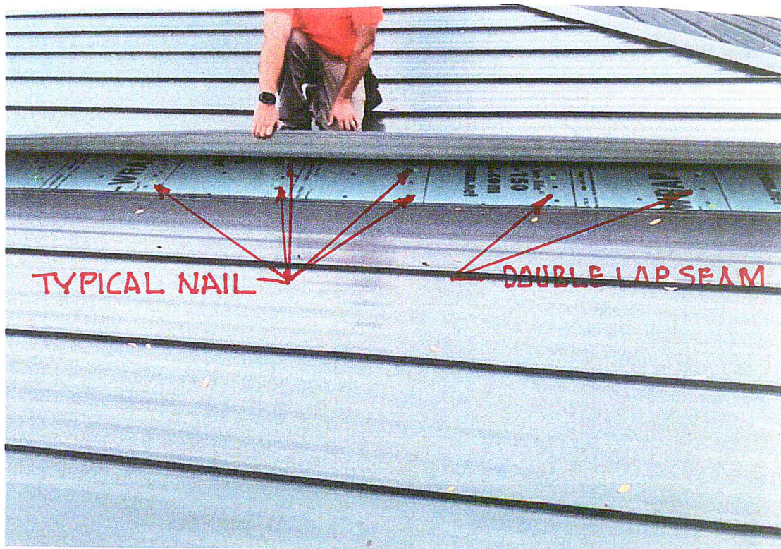
UNDERLAYMENT INSTALLATION
