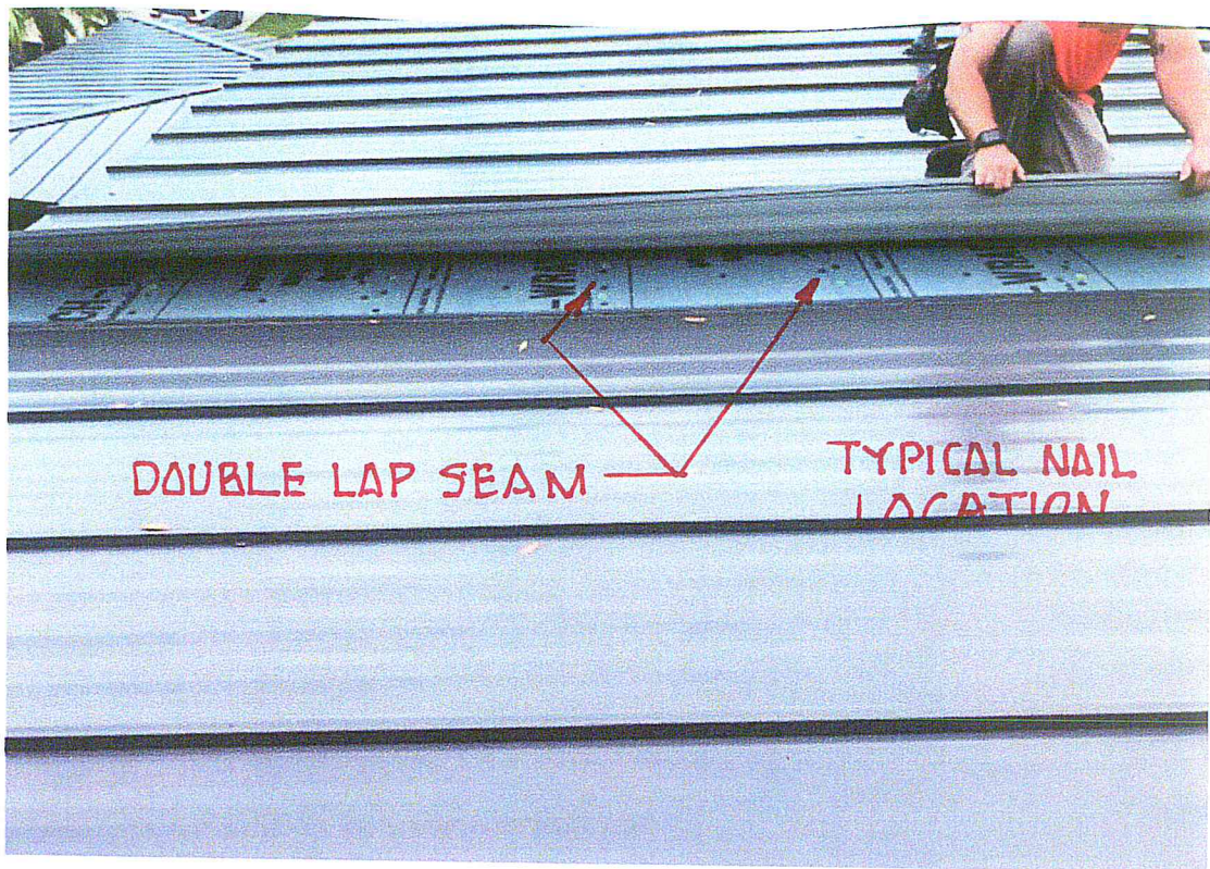
UNDERLAYMENT INSTALLATION
